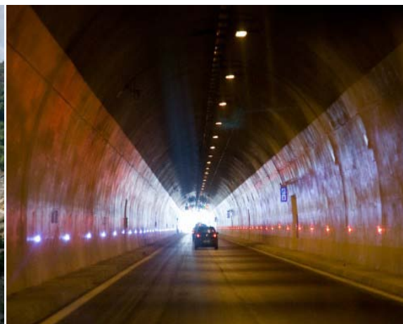
Fig. III.13 Tuneli i Elbasanit
